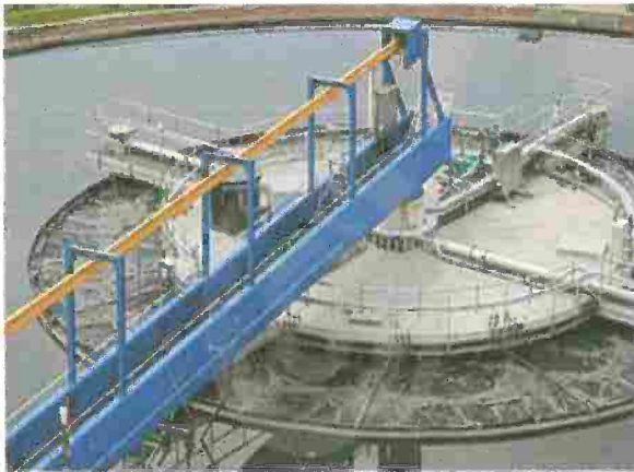
White Tanks Regional Water Treatment Facility
